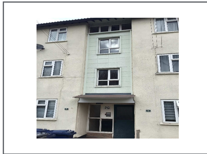
Photo 6 – Ekin Road Block – Front Entrance
