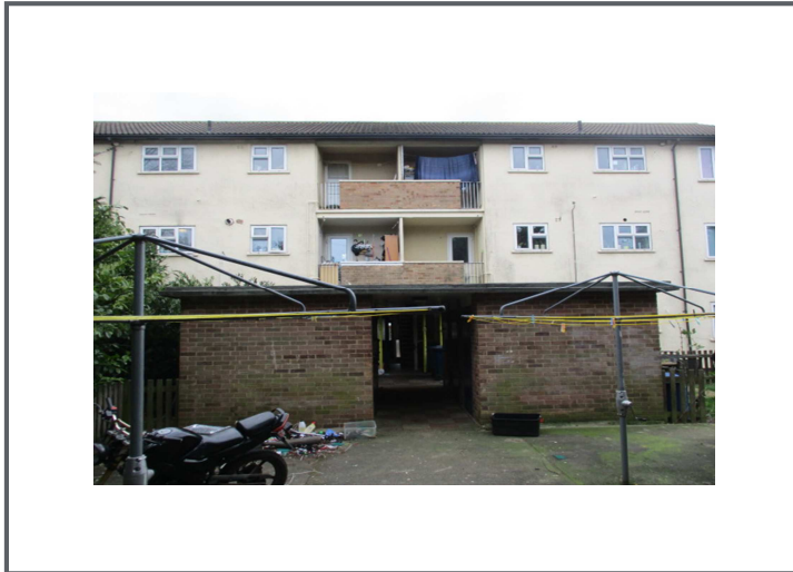
Photo 3 – Ekin Road Block Rear Elevation
