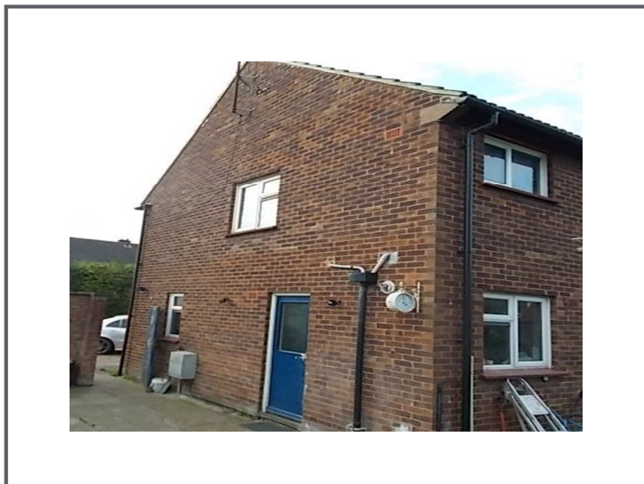
Photo 13 – Ekin Road House –Gable Elevation
