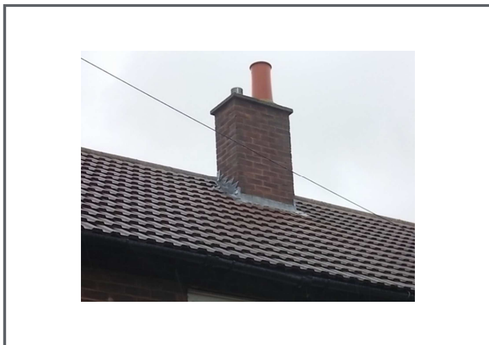
Photo 15– Ekin Road House – Roof Slope (Front)
