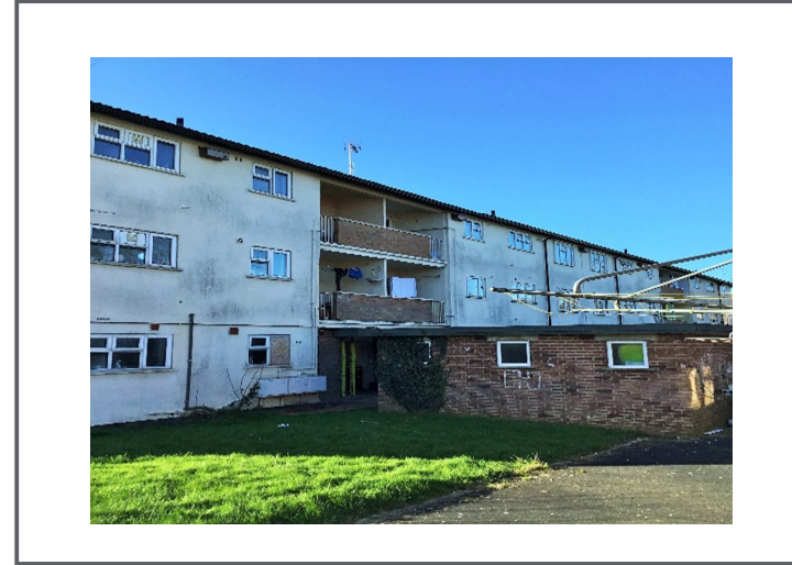
Photo 4 – Ekin Road Block Rear Elevation
