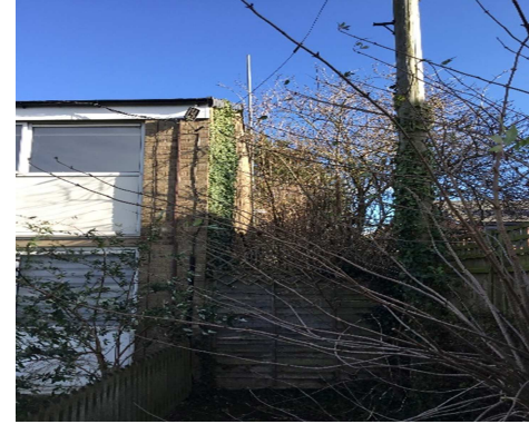
Photo 26 – Ekin Walk - Gable Elevation (Ivy)
