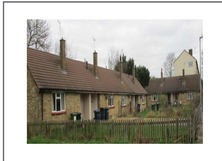
Photo 18 - Ekin Road Bungalows
