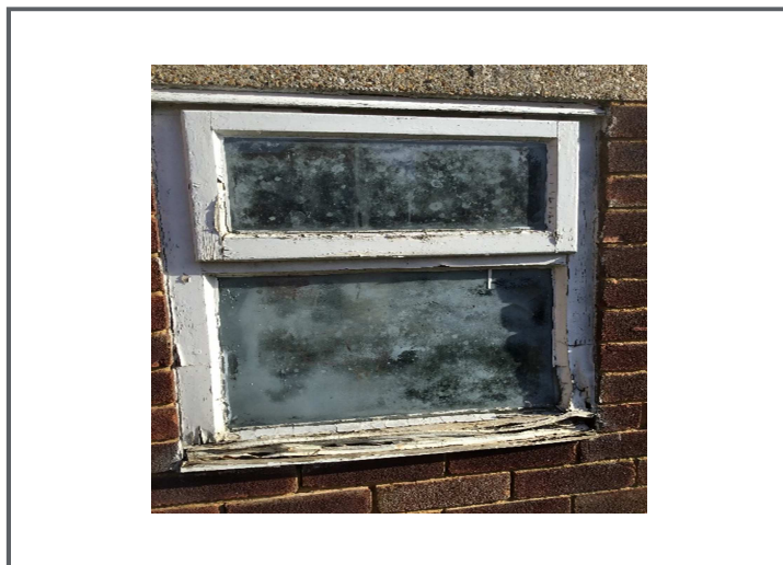
Photo 17 – Ekin Road Block – Shed Window
