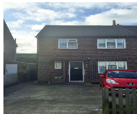
Photo 12 – Ekin Road House - Driveway
