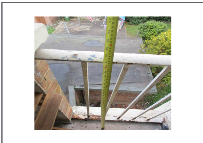
Photo 7– Ekin Road Block – Rear Balcony Balustrade
